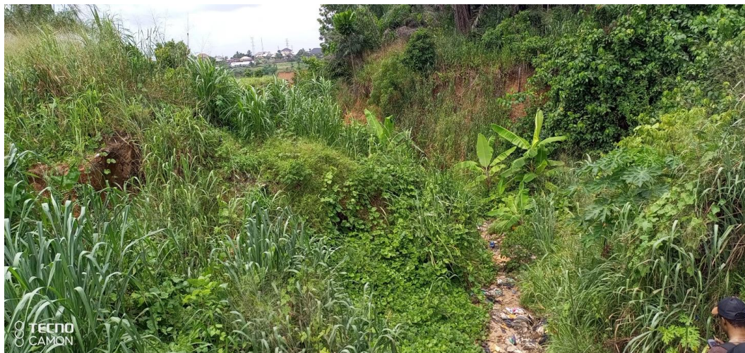
Fig 5: Gully erosion site at old nekede road owerri.
